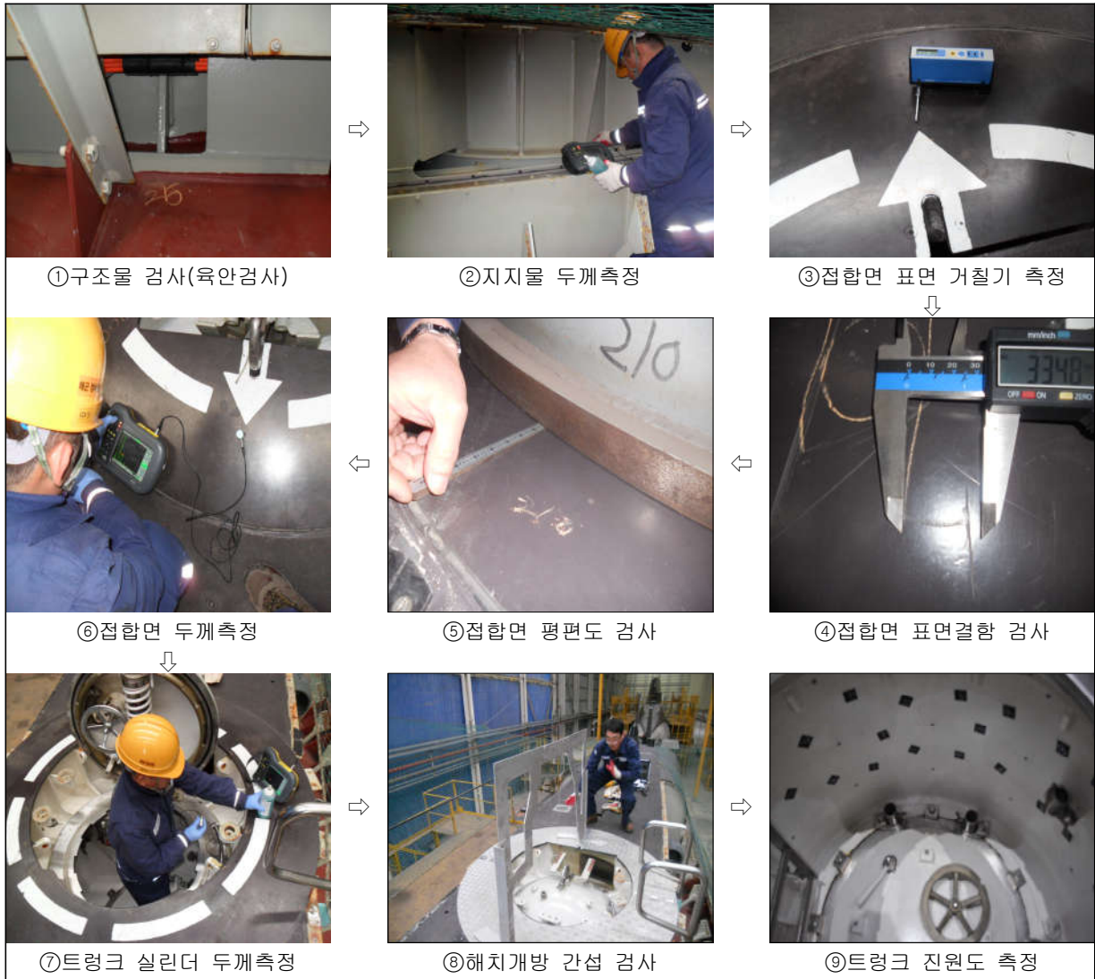
Fig. 5. Submarine Rescue Hatch Area Inspection Procedure
